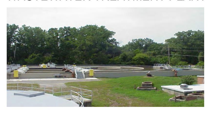
The Milan WWTP was upgraded in 2007 by Tetra Tech Engineering from a Rotating Biological Contactor plant to an Oxidation Ditch facility.
